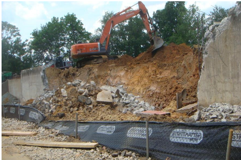
Figure 1: Large Retaining Wall Demolition
