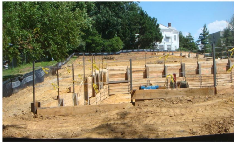
Figure 4: Material Storage/ Staging Area
